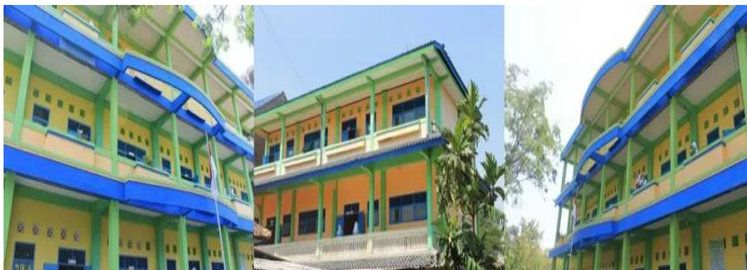
Figure 1. Research Location at MTs Sholihyyah Kalitengah
