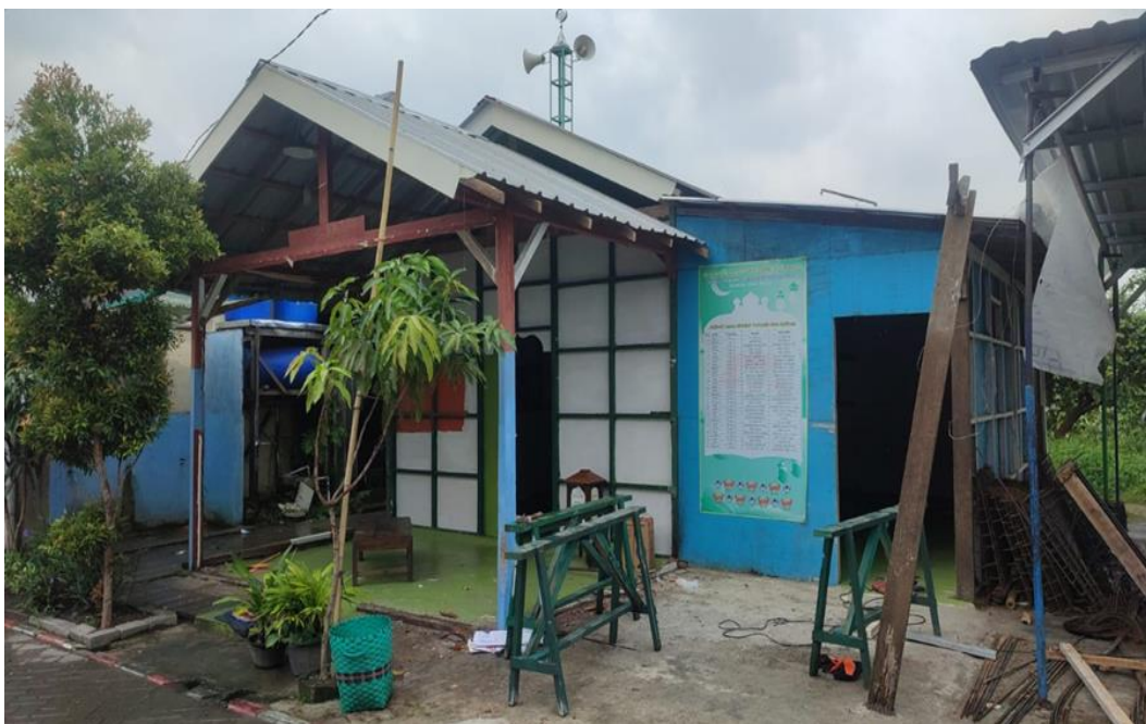
Figure 1. Mosque Darussalam Griya Salam Before Being Dismantled
